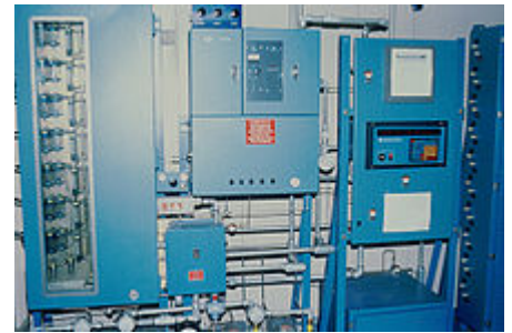
Pictured is a sophisticated gas chromatography system. This instrument records concentrations of acrylonitrile in the air at various points throughout the chemical laboratory
